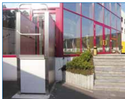
Platform lift at upper landing, providing access to commercial premises
