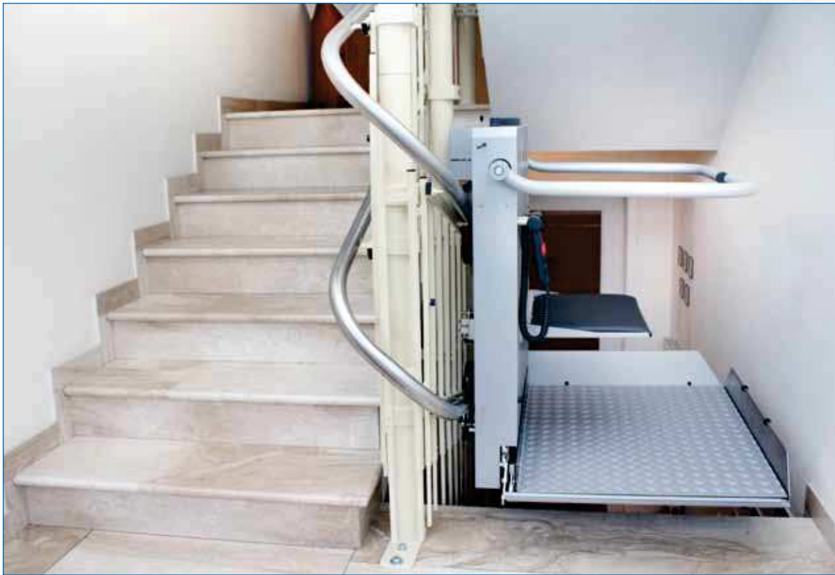
HIRO 320 with folding seat (optional equipment), with guide rails on posts in the stairwell
