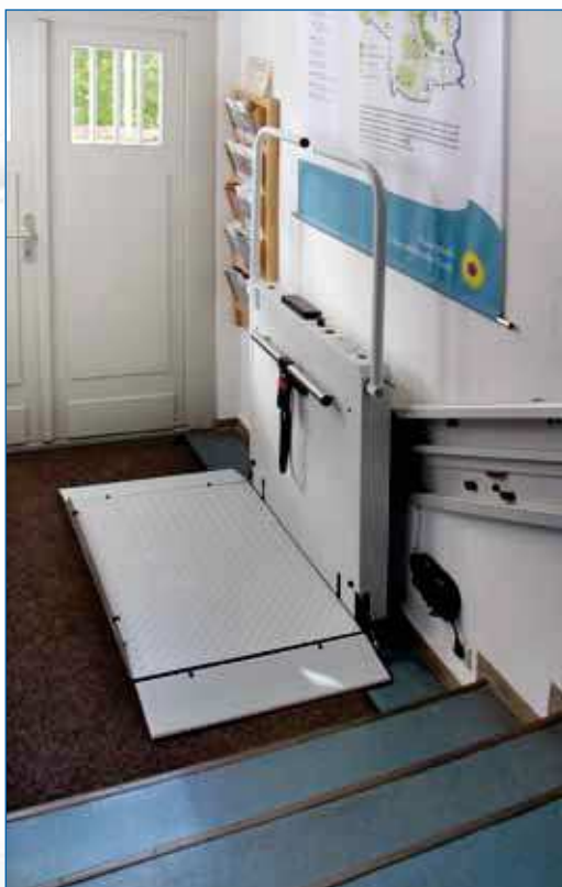
Wall-mounted installation of a HIRO 350
